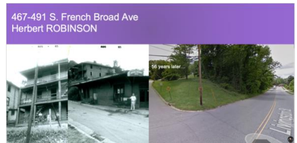
Fig. 4. Before and after urban renewal (1969 to 2021): B53-P1
